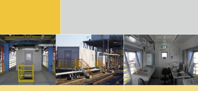
Electrical/instrumentation, operation and CO<sub>2</sub> extinguisher containers
